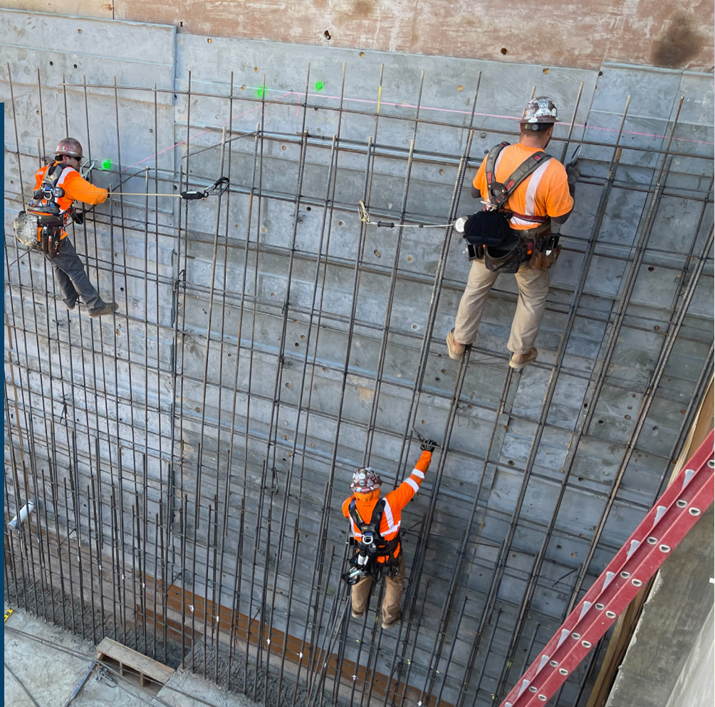
Photo: Construction of the Ventura Street Undercrossing
