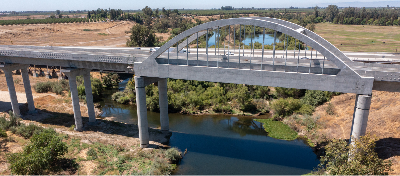
Photo: San Joaquin River Viaduct
