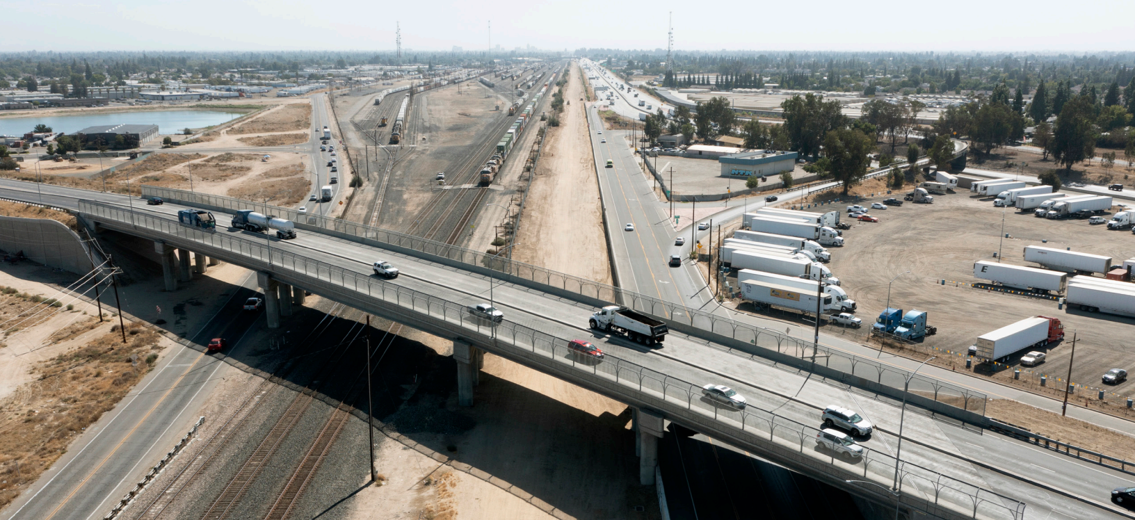
Photo: Ashlan Avenue Viaduct
