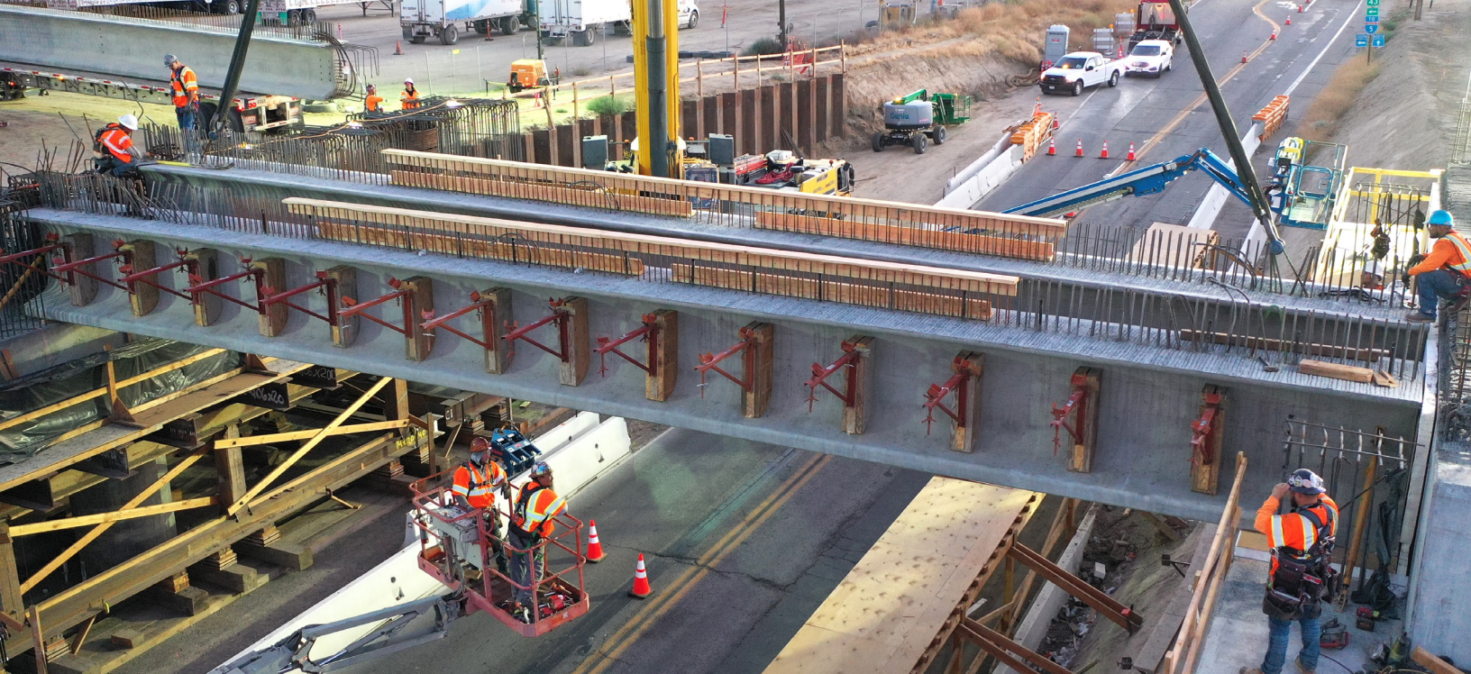
Photo: State Route 46 Overpass
