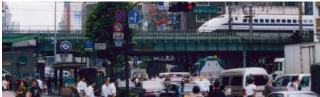
Figure 2.3 Shinkansen on elevated track travels through Tokyo
