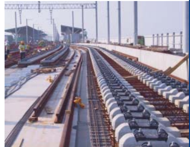
Figure 3.5 Laying tracks, Taiwan, ROC
