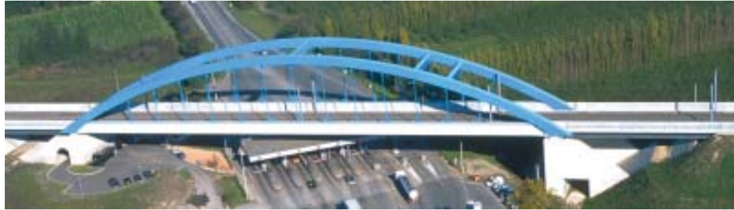
Figure 2.2 TGV Mediterranean line crosses A7 toll plaza near Avignon
