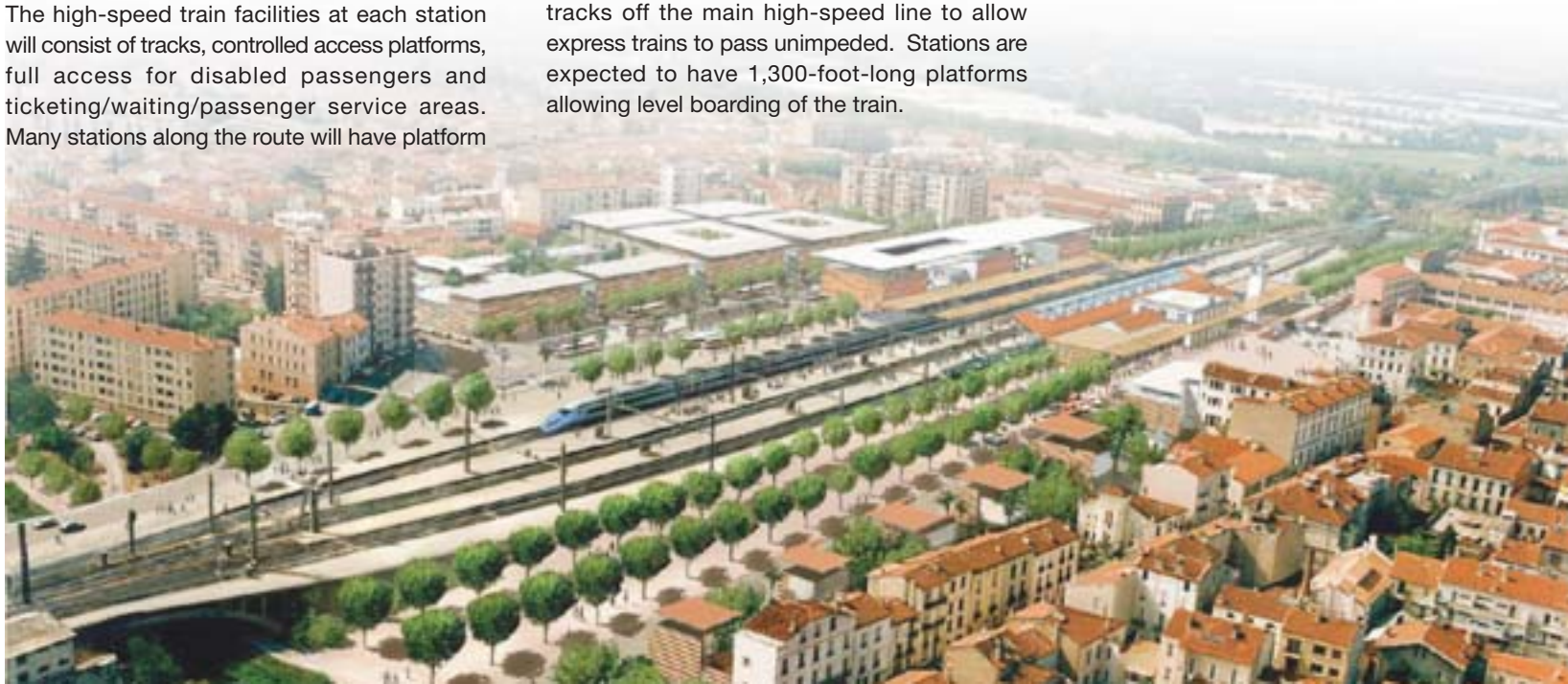
Figure 2.13 New TGV station and development at Perpignan
