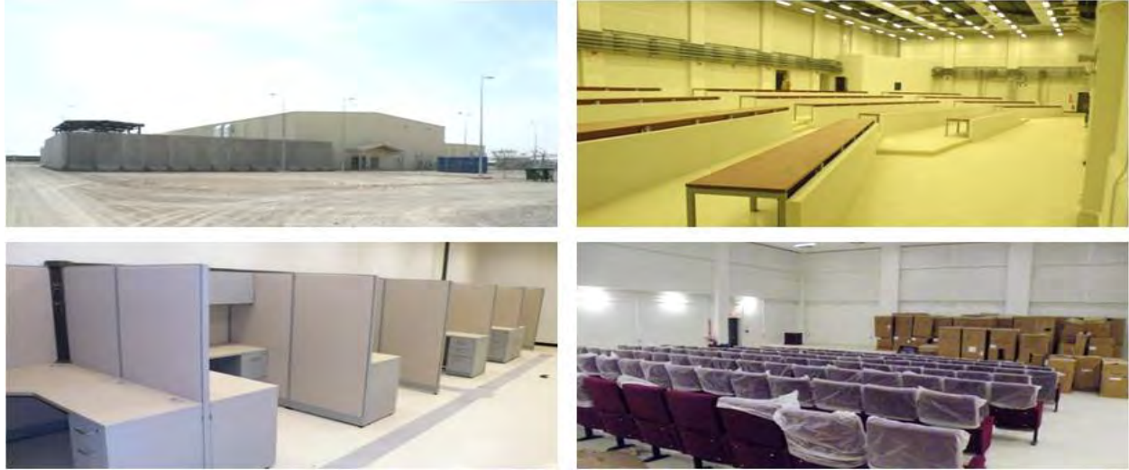
Figure 1 - Photos of the 64K building during a site visit on May 8, 2013. Top left: exterior view; top right: tactical operations center; bottom left: cubicles; bottom right: unopened boxes and unused chairs. (Source: SIGAR)
